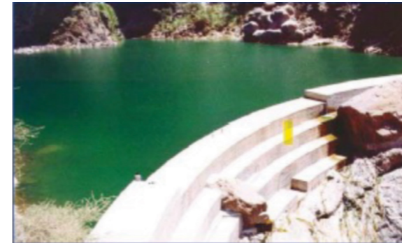
Figure 37: Surface Storage dam.
